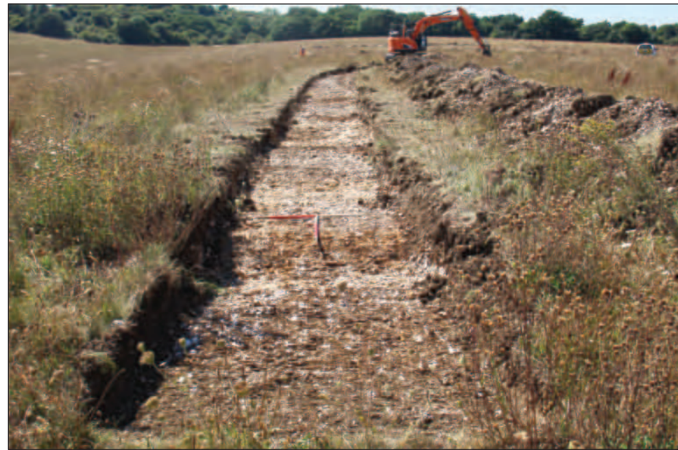
Trench 69, looking west (1m scales)
