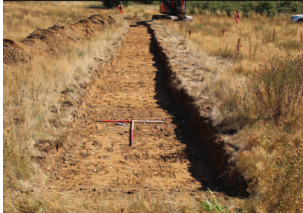
Trench 58, looking north-east (1m scales)
