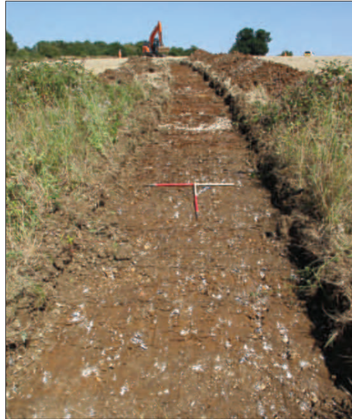
Trench 107, looking north-west (1m scales)
